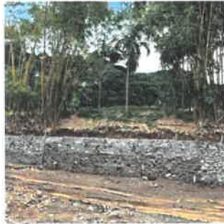
REPAIR OF RIPRAP
