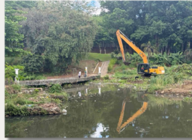
LAGOON AND RIVER DESILTING WORKS
